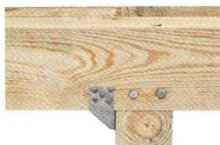
Skid End Double Lag-Bolted and Hurricane Clipped
