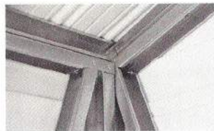
Roof Connection to Side and End Wall
