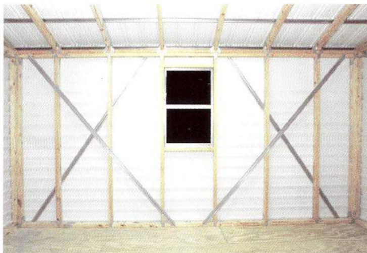
Shear Wall Bracing
