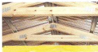
Roof Assembly with Steel Hat Channel
