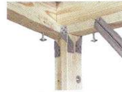
Corner Bolt Connection on Vaulted Wall Building
