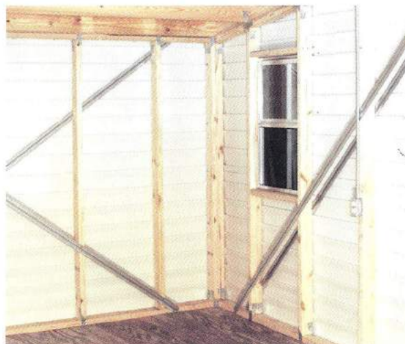
Vaulted Wall & Roof System
