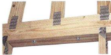
Bolt Connection to Double Top Plate
