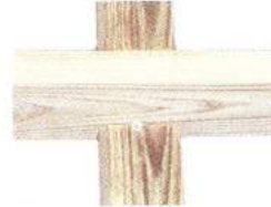
4" Lag Bolt Connecting Crossmember to Skid
