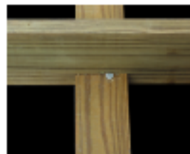
2x6" Floor Joist Connected to Skid with 4" Lag Bolt
