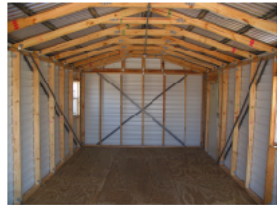
Roof Joist with Collar-Tied Truss Plate Connections
