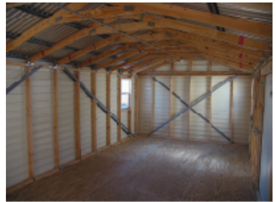
Rectangular Wall Sections with T-Wall Bracing
