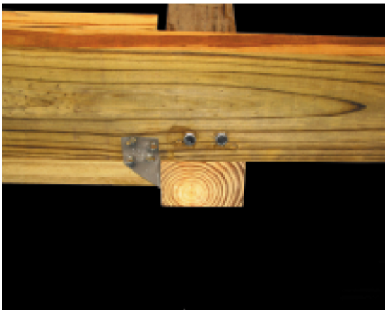
Skid End Double Lag-Bolted and Hurricane Clipped
