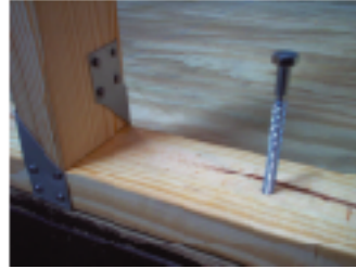
4" Lag Bolt Connection on Wall Bottom Plate to 2x6" Cross-member
