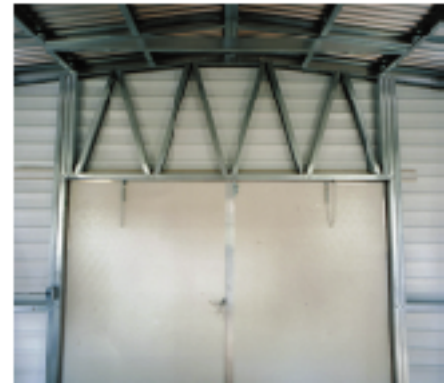
Diagonal Double Door Support
