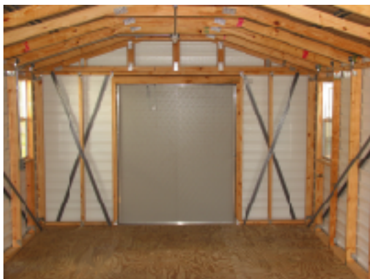
Shear Wall Bracing with 60" End Door
