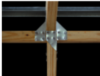
Triple Hurricane-Clipped Connection to Roof Rafter and Top Plate
