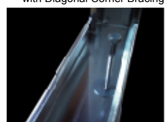
Accusteel 4" Lag Bolt with Washer - Bottom Plate Connection
