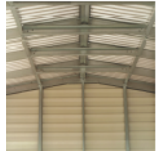
Accusteel Wall and Roof Structure
