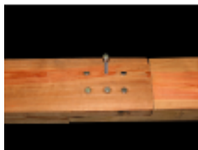
Skid Splice on 4x6" with 4" Lag Bolt Connection
